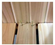
**Step 5:** Position Corner Caps on top of Legs and center on leg. Caps hang over outside of leg roughly 3/4 of an inch. Fasten with **Small** screws using pre-drilled holes. DO NOT OVER TIGHTEN
