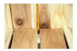
**Step 5:** Position Corner Caps on top of Legs and center on leg. Caps hang over outside of leg roughly 3/4 of an inch. Fasten with **Small** screws using pre-drilled holes. DO NOT OVER TIGHTEN
